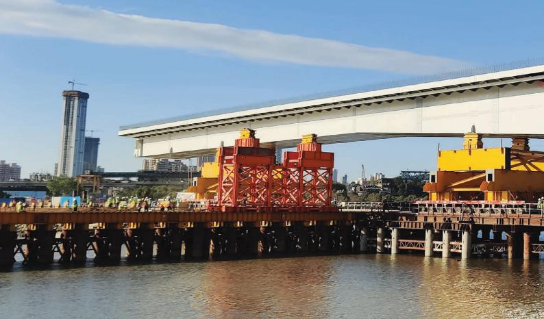
Express Global Logistics (EXG) moving an orthotropic steel deck, weighing 1,362 tonnes, in Mumbai.
